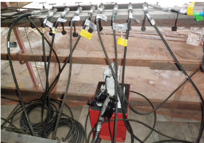
Below: 8-point manual manifold lift system
